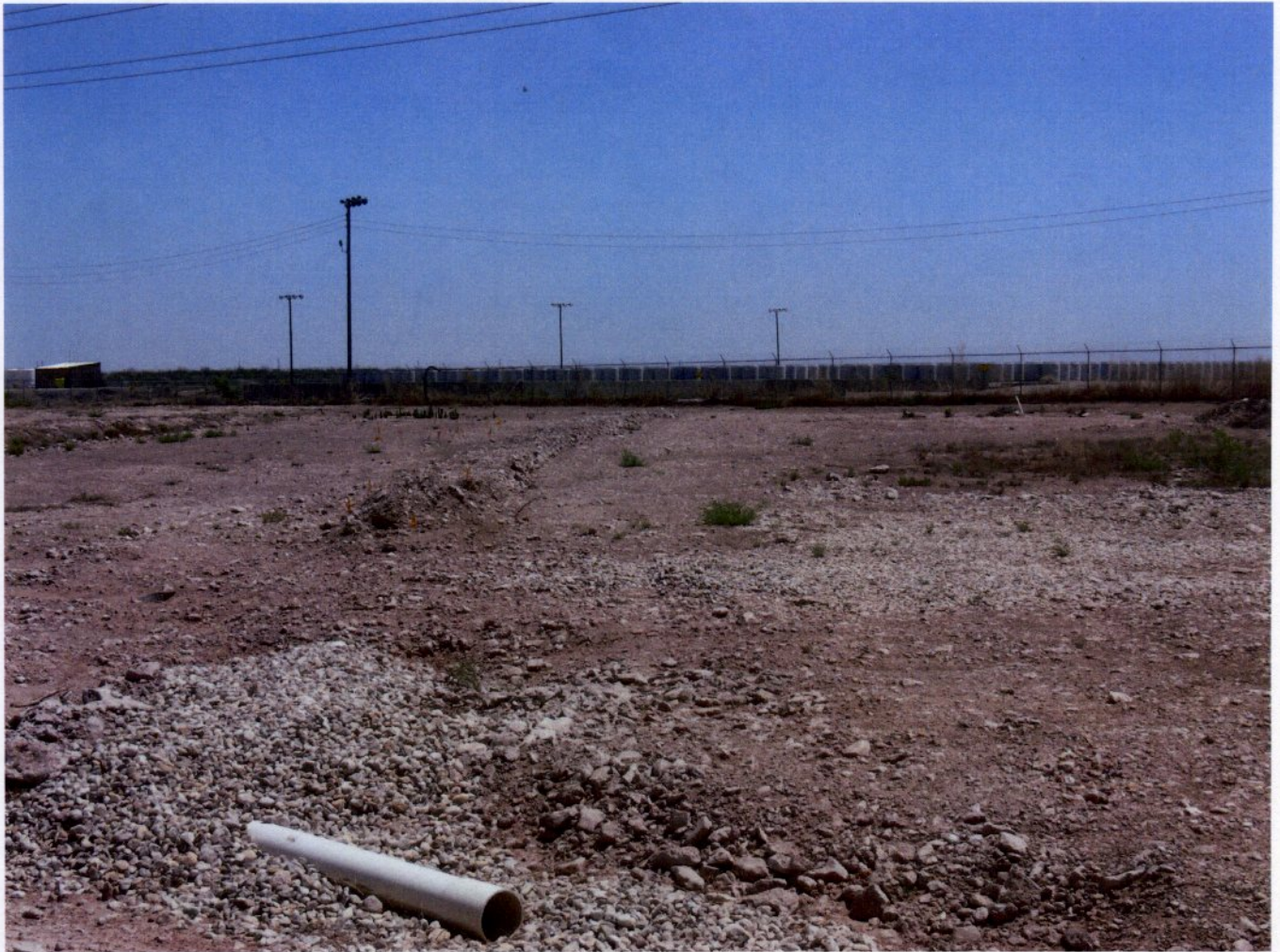
Figure 5 Drainage diversion pipe from LSA pad to state line road. This pipe was installed to move runoff water from the pad away from the area around OAG monitor well TP-42, as required by License Condition 41.
